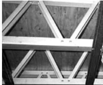
Figure 7: Typical lightweight fabricated steel joists
