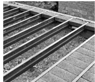
Figure 10: Typical concrete beam and block floor
