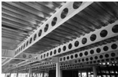
Figure 8: Typical lightweight cellular steel joists
