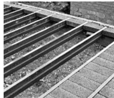
**Figure 10:** Typical concrete beam and block floor
