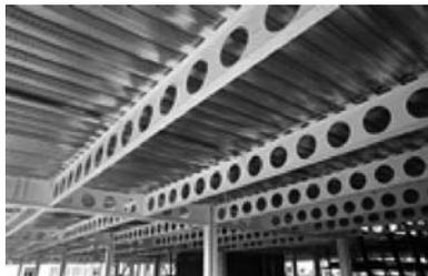
**Figure 8:** Typical lightweight cellular steel joists
