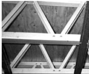
**Figure 7:** Typical lightweight fabricated steel joists
