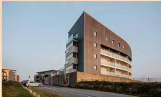
Designed using an uncompromising contemporary approach, Fistral Blue employs a varied pallet of quality materials – copper, stone, glass and render – detailed in a crisp and simple fashion. Copper cladding is finished in an oxide brown patina chosen to complement the colours and hues of the natural coastal locale, and the texture and colouring of the neighbouring Victorian brick-built Headland Hotel.
