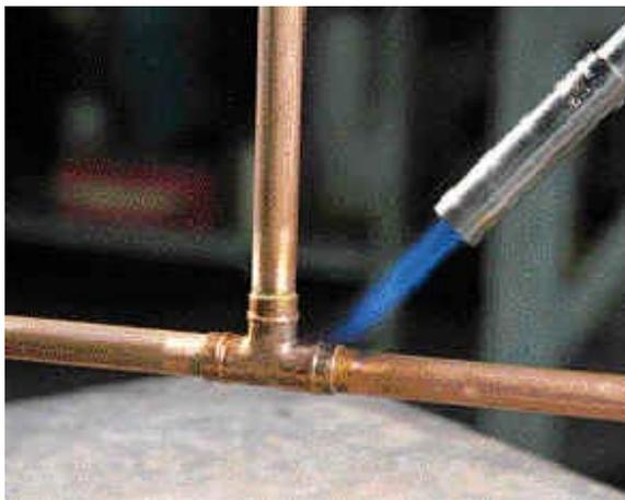
*Figure 10 – Heating the joint, integral solder ring fitting*
