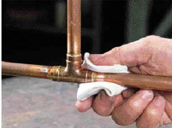
*Figure 12 – Removal of excess flux*
