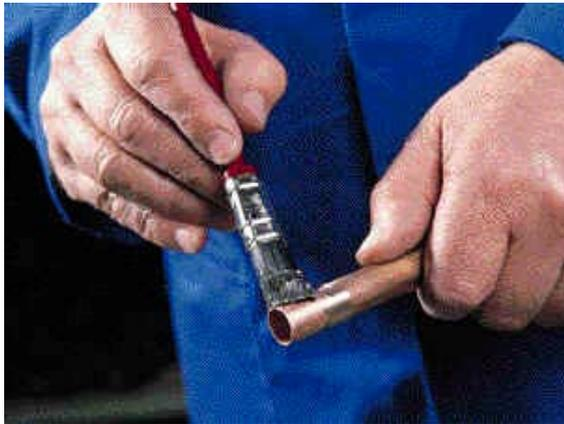
*Figure 8 – Applying flux to the tube end*
