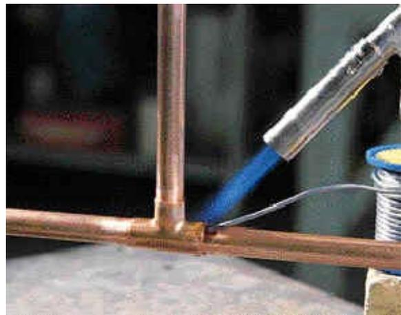
*Figure 11 – Heating the joint, end-feed fitting*
