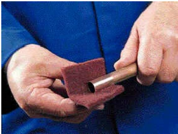
*Figure 6 – Cleaning the tube end*
