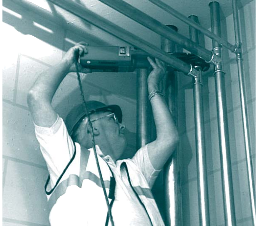
The new press fitting tool in action. The picture demonstrates the speed and ease of installation.
