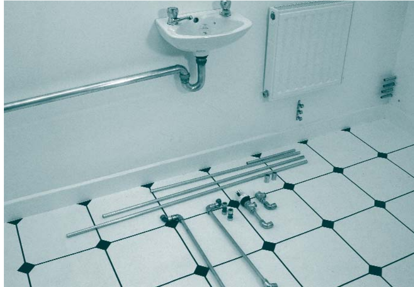
Push-fit fittings are ideal for making final connections as demonstrated in above and opposite pictures.
